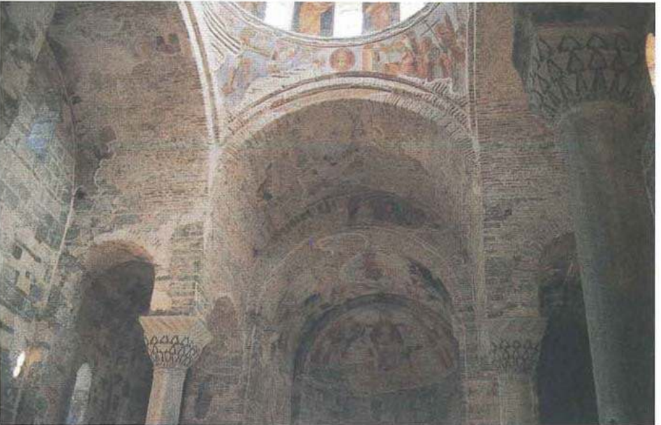
III General view of the interior of Hagia Sophia. east, looking towards the apse
